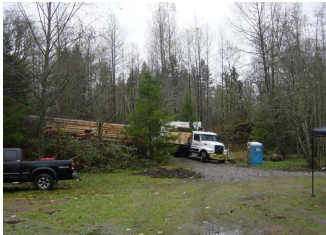
Arrival at Jobsite
