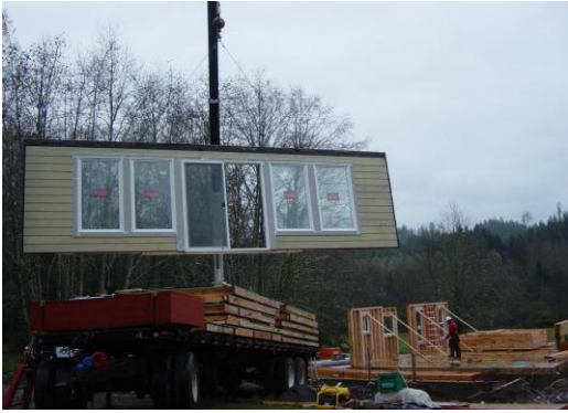
Complete wall lifted from the truck
