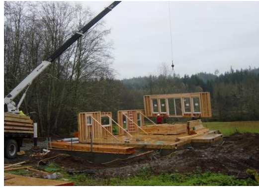
And being set in place
