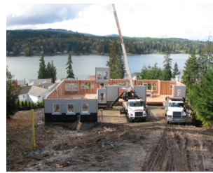
On-site while a framing package is being set by crane...
